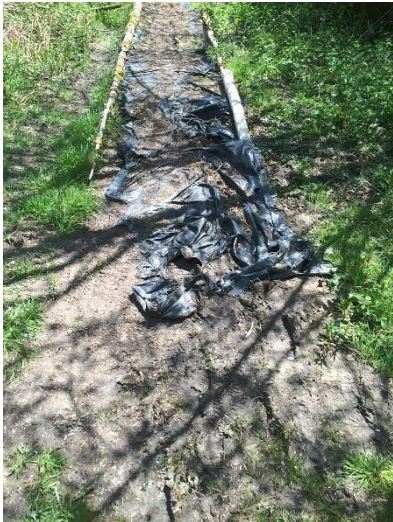
← Damage to path
